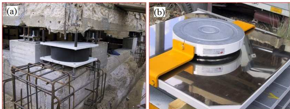
Fig. 2. (a) High damping rubber bearing (HDRB) and (b) low friction sliding bearing (LFSB) of the Solarino building.
