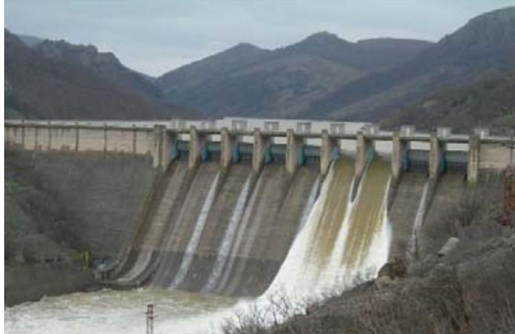
Fig. 1: Dam with typical control elements at the top (Picture: D. Kisliakov).
